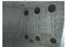
The Century-Line Sleeves await the pipe and Link-Seal modular seals, for the no leak solution in this pump room. Please notice that the 24" Century-Line Sleeves were no problem to install at the top of the wall. Contractors easily installed the Century-Line Sleeves; steel sleeves would have been a heavy load to install at this height.
